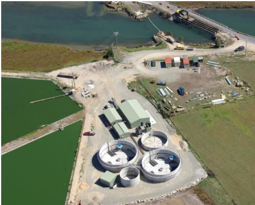
Figure 4: The St. Helens WWTP during construction
